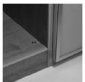
Adjustable feet are placed under each base to ensure the stability and the vertical and horizontal alignement of each element over the time.
